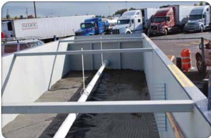
Internal view of Aquip, adjacent to truck parking area
